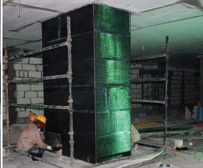
section of the element. Jacketing involves fixing of additional reinforcement, shuttering and pouring micro concrete. This is not only a tedious and time consuming method, but also results in reducing clear span or reduced carpet area. Steel plates are likely to corrode over a period of time. Also it is difficult to apply plasters and renders over steel plates. Both the above methods result in increased dead load over the existing structure.
