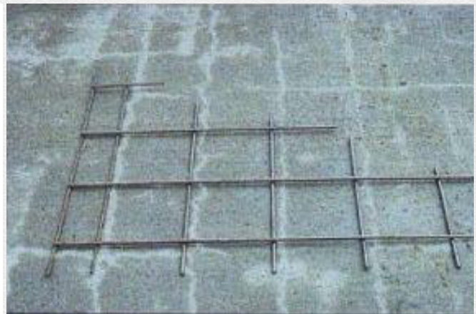
Figure 04. (Steel Mesh on Slab Surface)
