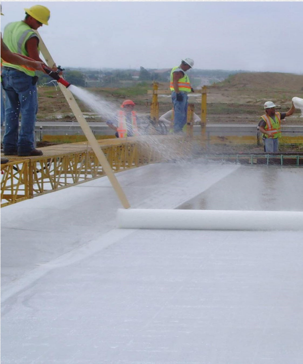
Proper Curing—immediate covering of Polythene Sheet , wet burlap (hessian cloth) and watering. (Fig. 05 & 04)
