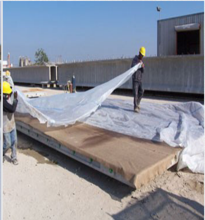
Proper Curing—immediate covering of Polythene Sheet , wet burlap (hessian cloth) and watering. (Fig. 05 & 04)
