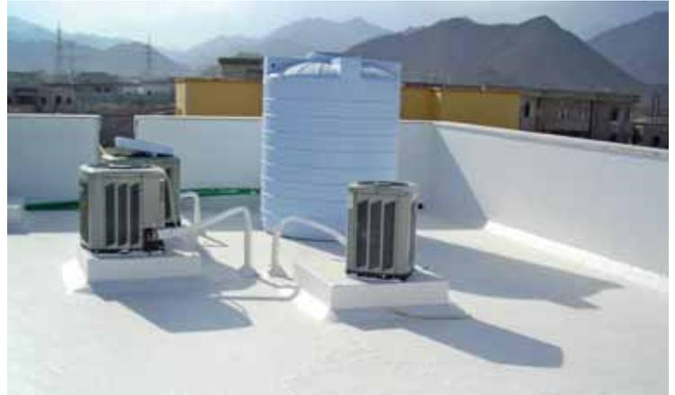
environment. Another single component, flexible, cold applied liquid water proofing membrane is MoyaShield PU. It is an extremely flexible membrane with elongation exceeding 500%.
